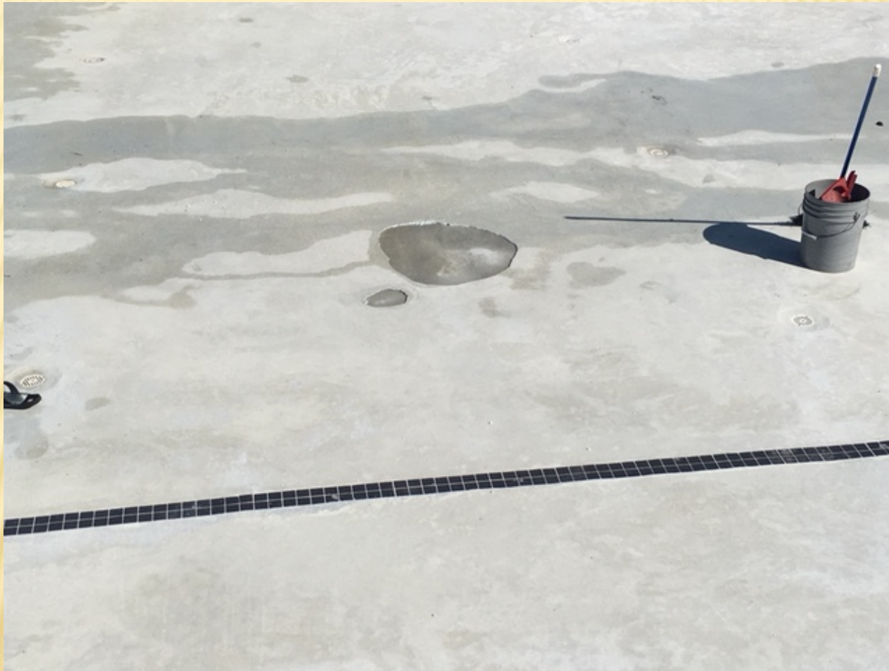
Bottom of pool showing delamination of marcite coating
